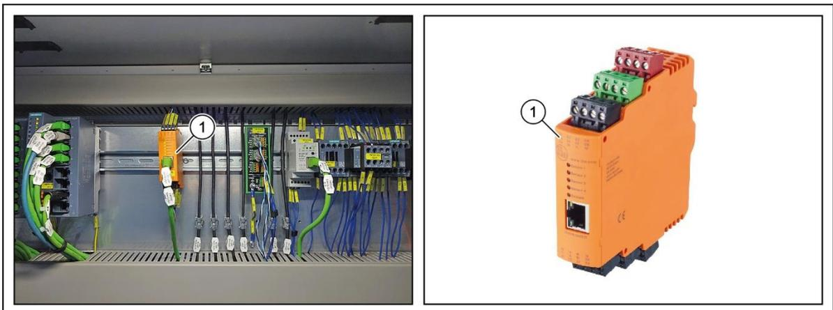
Fig. 107 VSE evaluation unit in the control cabinet
